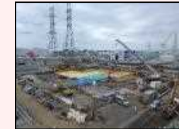
After dismantling in H1 east area
